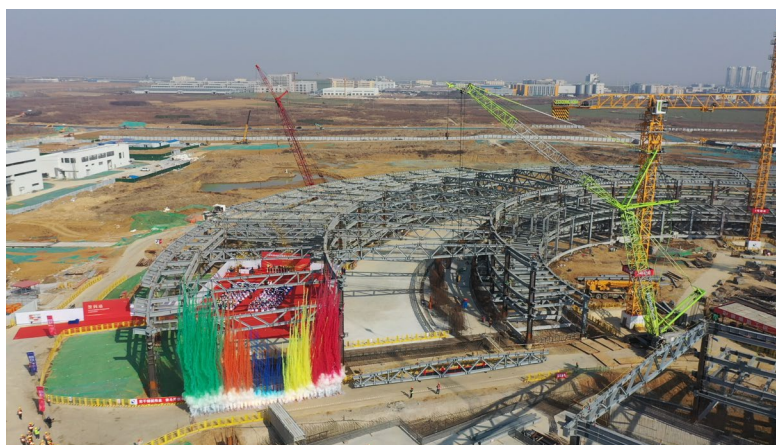
FIGURE 1. Hefei Advanced Light Facility (HALF) under construction, in Hefei, Anhui.
